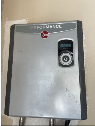
Rheem tankless water heater, model year is possibly 2020 though this is not confirmed with what was on the data sticker.
