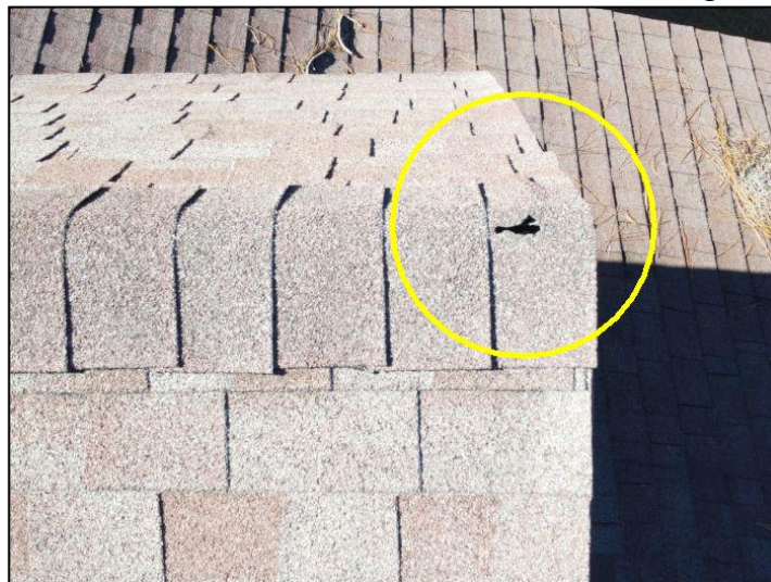
Some areas of the ridge to the dormers were damaged.
