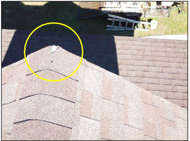
Some areas of the ridge to the dormers were damaged.
