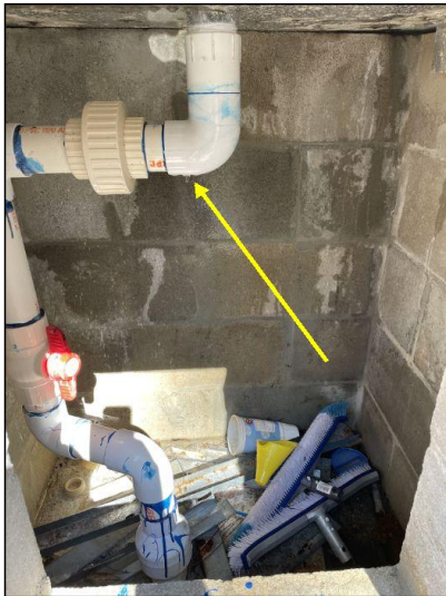
Water leak was observed inside the water fall feature enclosure.
