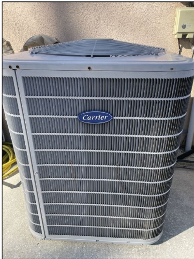
A/C unit, Carrier, model from 2010. 5 ton unit.
