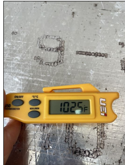
Due to the cooler ambient temperature outside, the heat was tested on the day of inspection. Satisfactory average. Pic of the air going out at evaporator coil.
