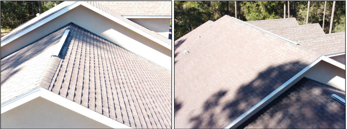
Overall views of the roof. Original to the home. 23 years old.
