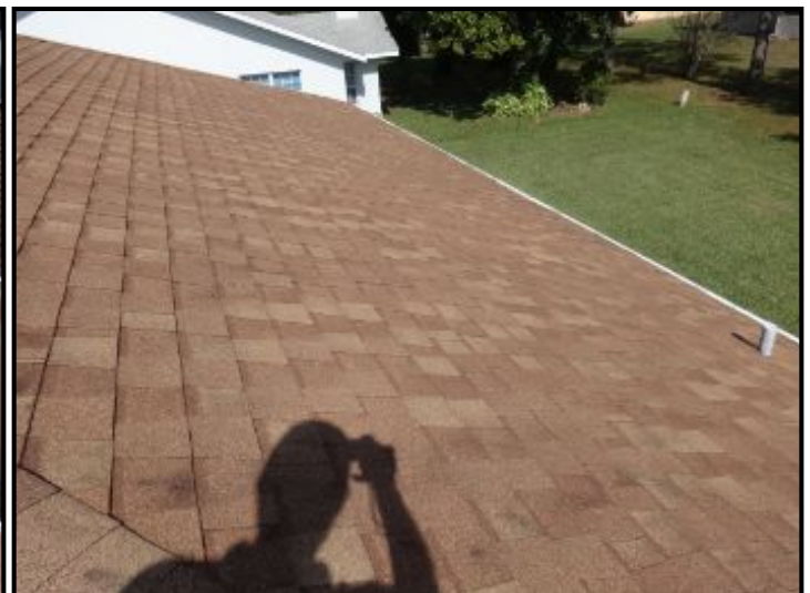
View of backside roof.
