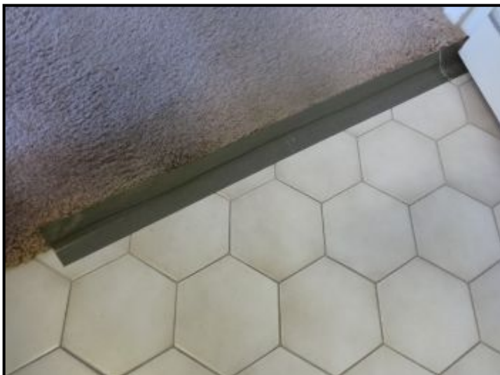
Tape used as a transition from the master bath to the bedroom.
