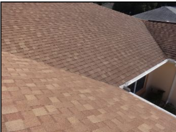
Front view of roof.
