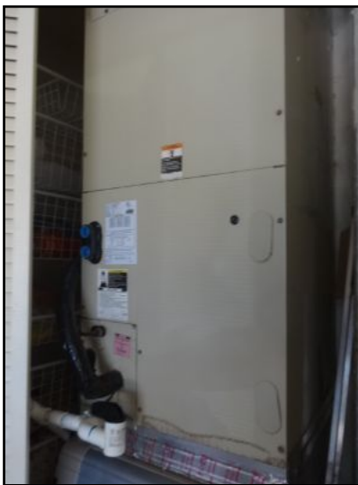
Air handler, Carrier, model from 2001
