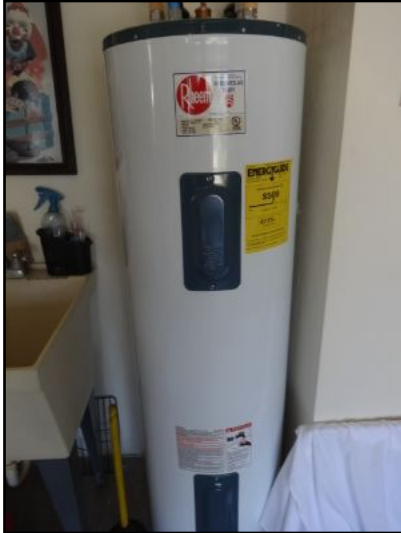
Rheem water heater, 40 gal, model year 2010.
