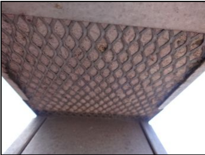
View of dryer vent on the roof. Recommend cleaning.
