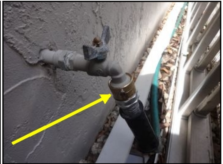
Example of an anti-syphon valve.
